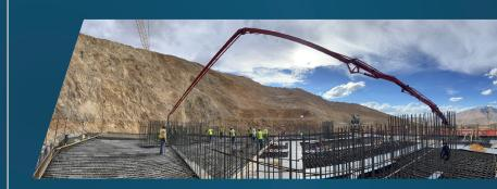
Malta Ready Mix was hired to supply concrete and equipment to the expansion project at the Rochester Mine. This expansion includes a new leach pad, a crushing facility equipped with two high-pressure grinding roll units, a Merrill Crowe process plant and "related infrastructure." Our team provided concrete with our batch plant and pumped concrete with our dedicated on-site pump truck.
